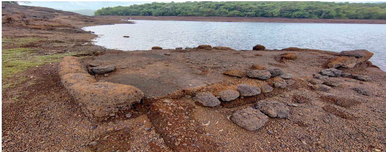
Fig. 4: The deteriorated house of curdi.
